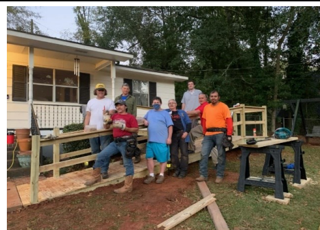
After the ramp was built safe access was accomplished.
